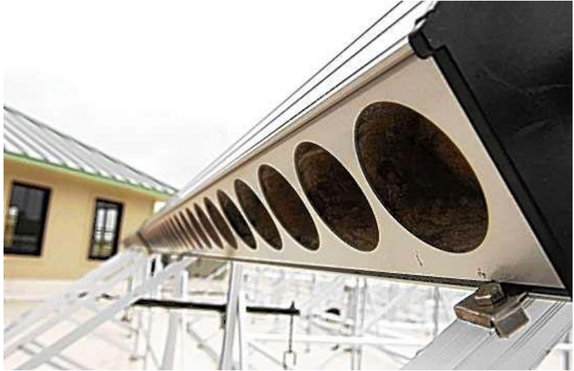
Ryan Prewitt photo - Solar evacuation tubes on Dardenne Prairie City Hall produce energy - not electricity - to run the city's geothermal heat pumps. Solar panels will produce 100 percent of the power for the city's heating and 30 percent of the cooling, and all the hot water needs.
